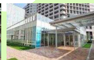
LAWSON hospital stores
