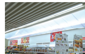
A sloped ceiling promotes natural ventilation, and the skylight introduces natural light.
