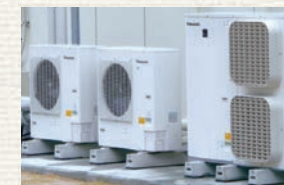
● Reduction of electricity consumption through use of CO 2 coolant
