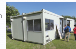
Prefabricated community space installed in the aftermath of the Kumamoto Earthquakes
