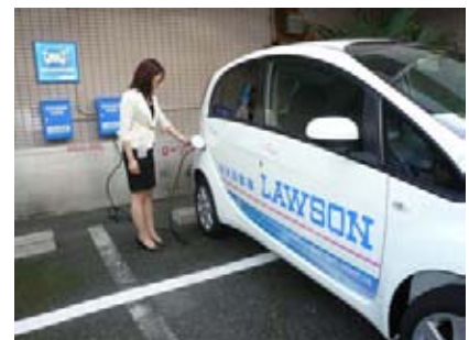
Some stores are being fitted with EV recharging points.
