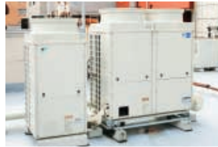
Exterior unit for integrated cooling and ventilation system
