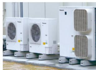
CO<sub>2</sub> refrigerant cooling/refrigeration system
