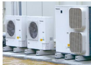
CO<sub>2</sub> refrigerant cooling/refrigeration system
