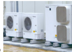
CO 2 refrigerant cooling/refrigeration system
