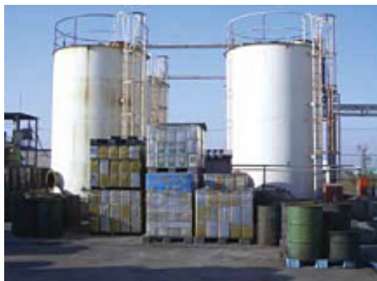
Waste oil recycling plant
