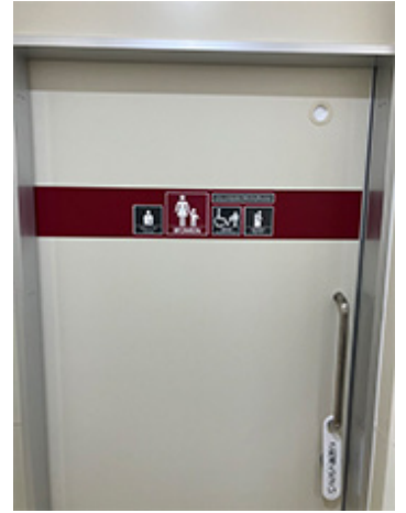
▲ A larger door has been installed to help customers enter the toilet.
